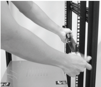
1. Secure the side rails to the rack.
